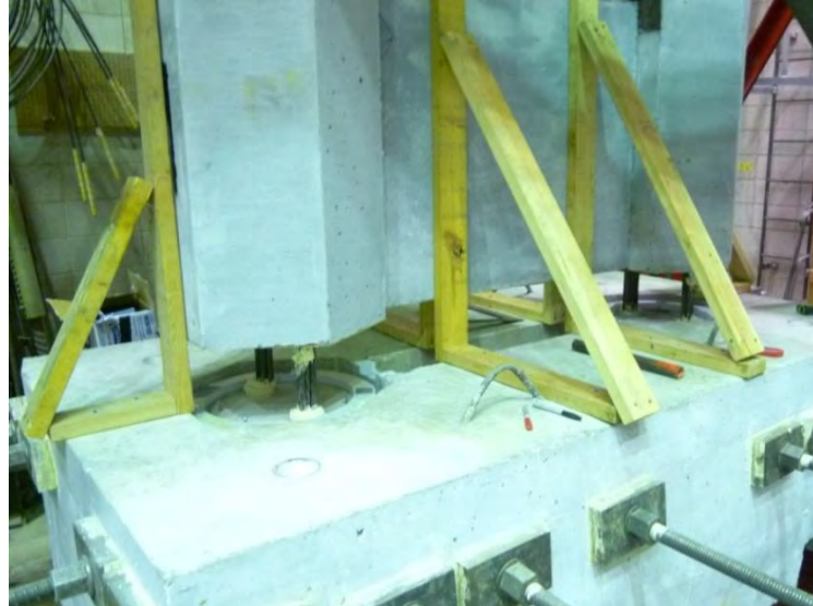
Figure 4.24: Placement of HCUP-BC Specimen on the Foundation Block
