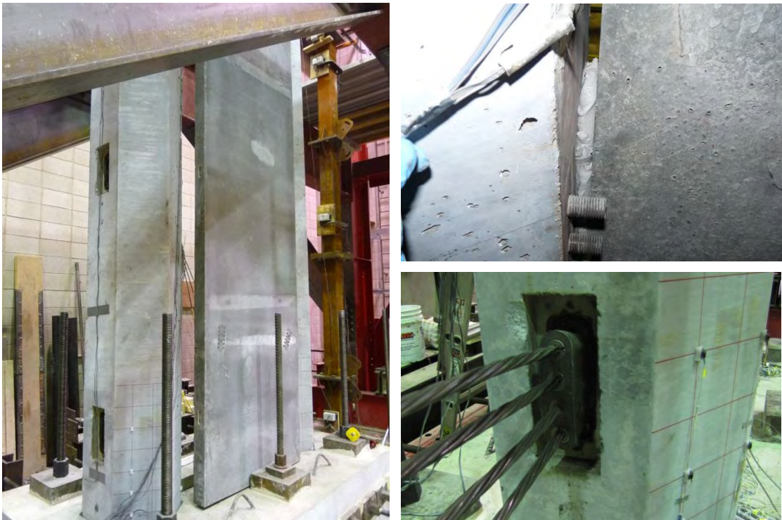
Figure 4.25: Placement of HCUP-HPT Panel and Interface Epoxy
