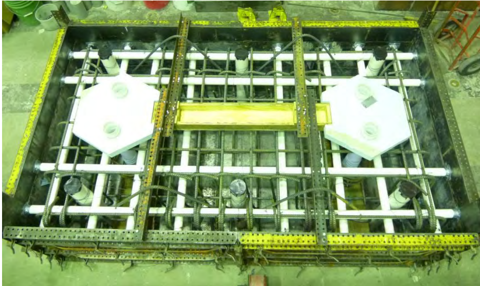
Figure 4.21: Foundation Block Formwork
