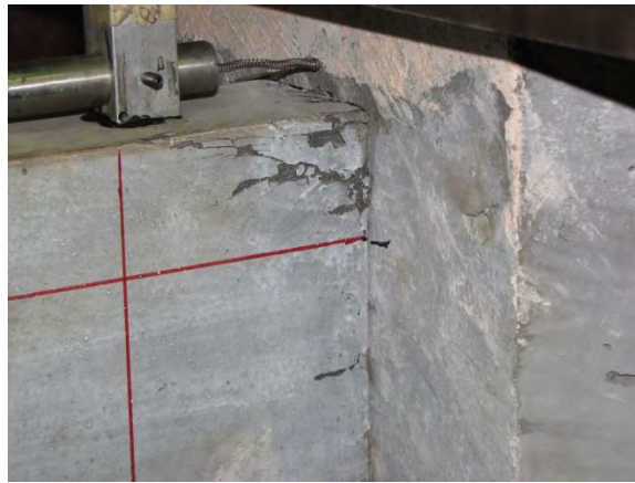
Figure 4.35: Localized Crushing at Top of HCUP-BC Panel
