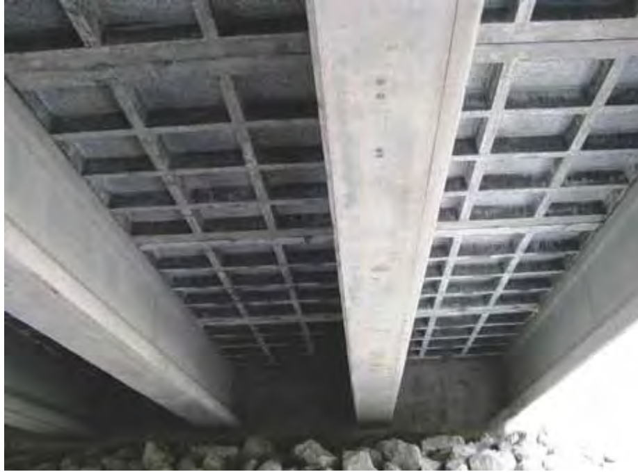
Figure 2.9: Underside of UHPC Waffle Deck Bridge (Moore, 2012)
