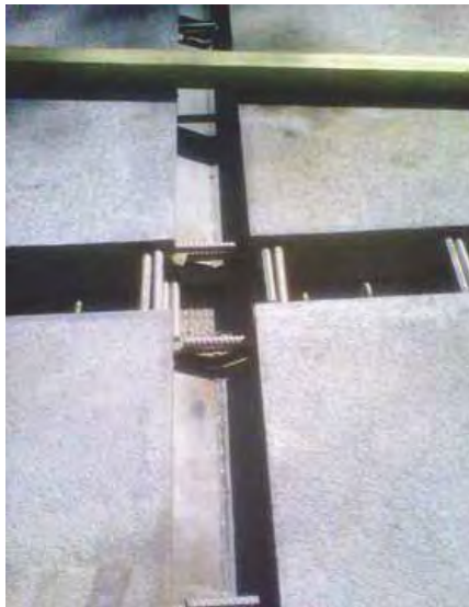
Figure 2.10: Construction Joints on Little Cedar Creek Bridge (Moore, 2012)
