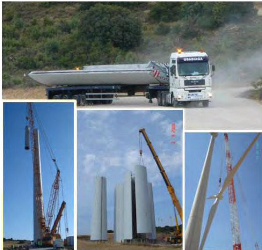
Figure 1.5: Transportation and Erection of Inneo Wind Tower (Grupo Inneo, 2008)
