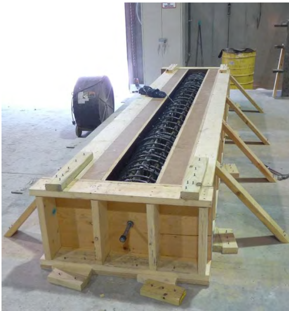
Figure 4.19: In-Plane Test Column Formwork
